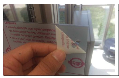
Peel back the protective film near each hole on the panel, just enough to uncover the hole.
